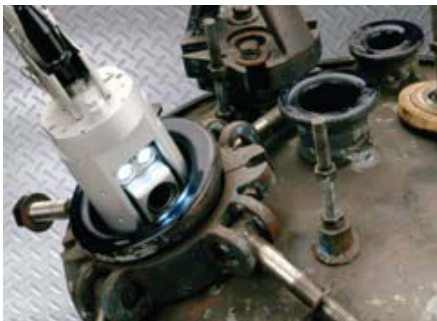
Inspection through a 100mm (3.94 in) \emptyset nozzle
