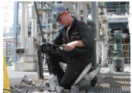
Tank and vessel inspection
